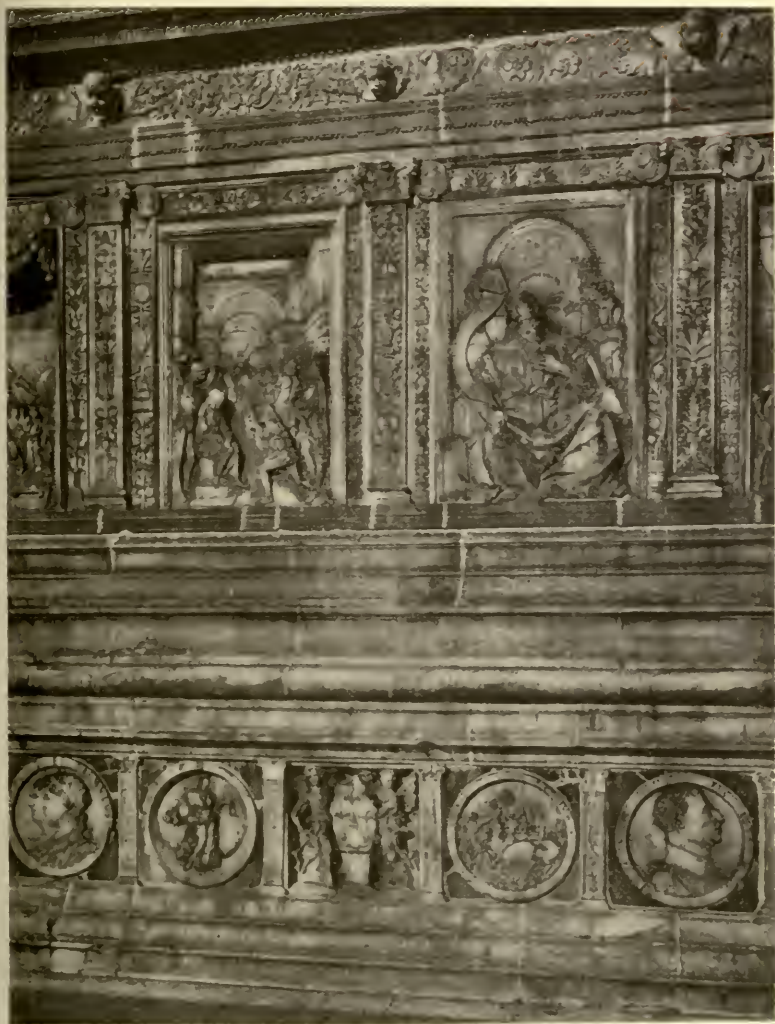
DETAIL OF FAÇADE Certosa, Pavia
